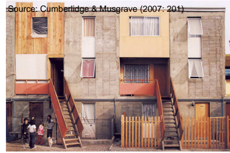
Source: Cumberland & Musgrave (2007: 201) QUINTA MONROY HOUSING PROJECT, CHILE
